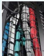
The steel wire frame provides the rugged support needed to manage the increased cable count and weight and provides airflow helping with heat dissipation.
