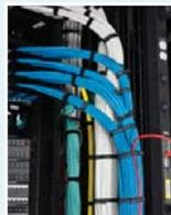
Category 6A Increased cable O.D. demands more room and provides support behind the rack to tie off and manage the abundance of horizontal cable being installed.
