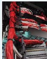
Increased port count necessitates a controlled cable management system to address the routing, management and administration of patch cords.
