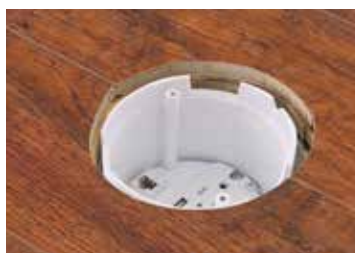
Wire devices into box
