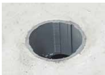
Cut box top level with concrete
